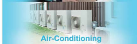
Air Condition Installation
