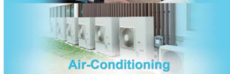
Air Condition Installation
